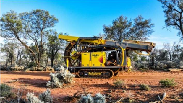
Coiled tube drill rig (MinexCRC, 2023)
