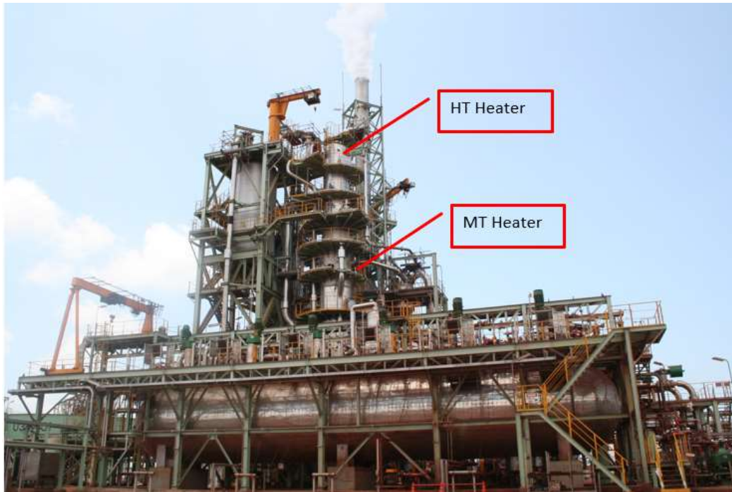
Figure 5 – Coral Bay Heater Train Arrangement
