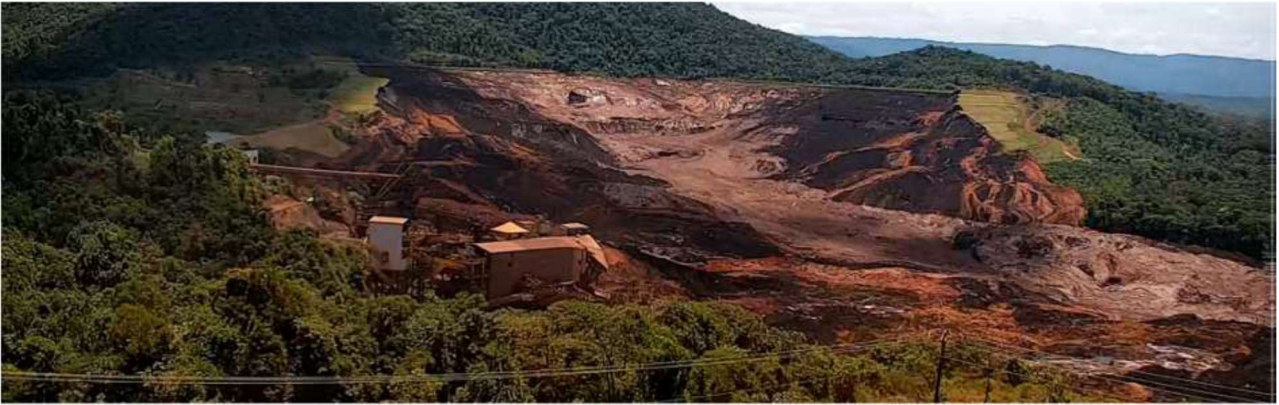
Figure 4 : Moments after the failure of Feijao Dam 1, Brumadinho (Ref (2))
