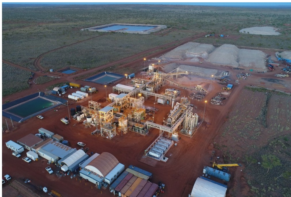
Figure 1 - Northern Minerals' Browns Range pilot plant
