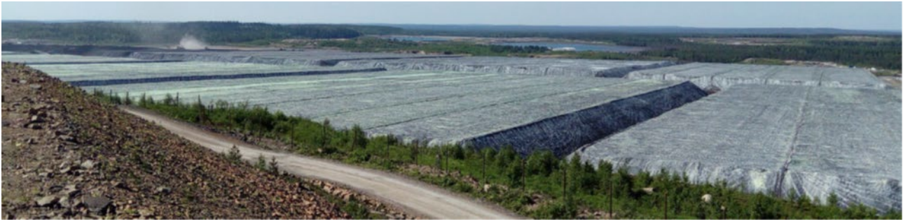
Figure 17: A panoramic view of the primary heap leach pad at the Talvivaara heap bioleaching plant
