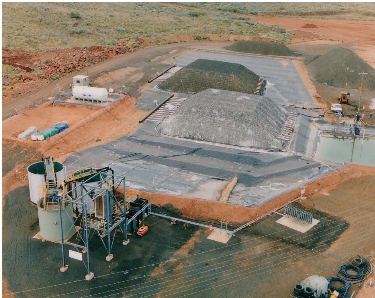
Figure 9: The 5,000 tonne BioHeap™ test heaps at the Mt Sholl/Radio Hill project (24)
