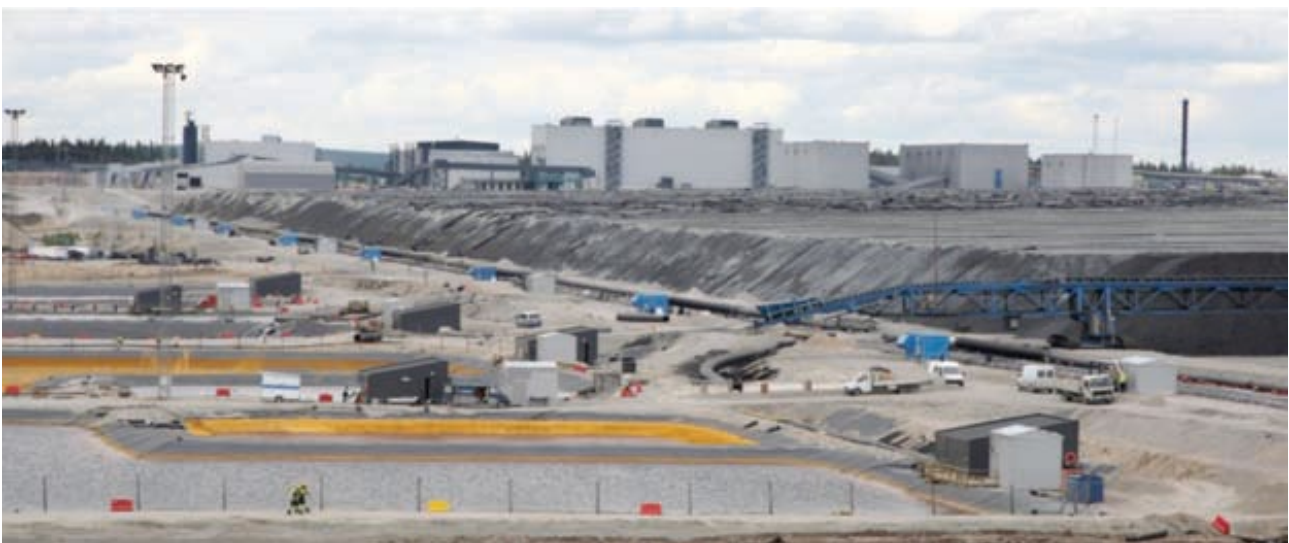
Figure 16: A view of the primary heap leach pad and the PLS ponds at the Talvivaara heap bioleaching plant (28)
