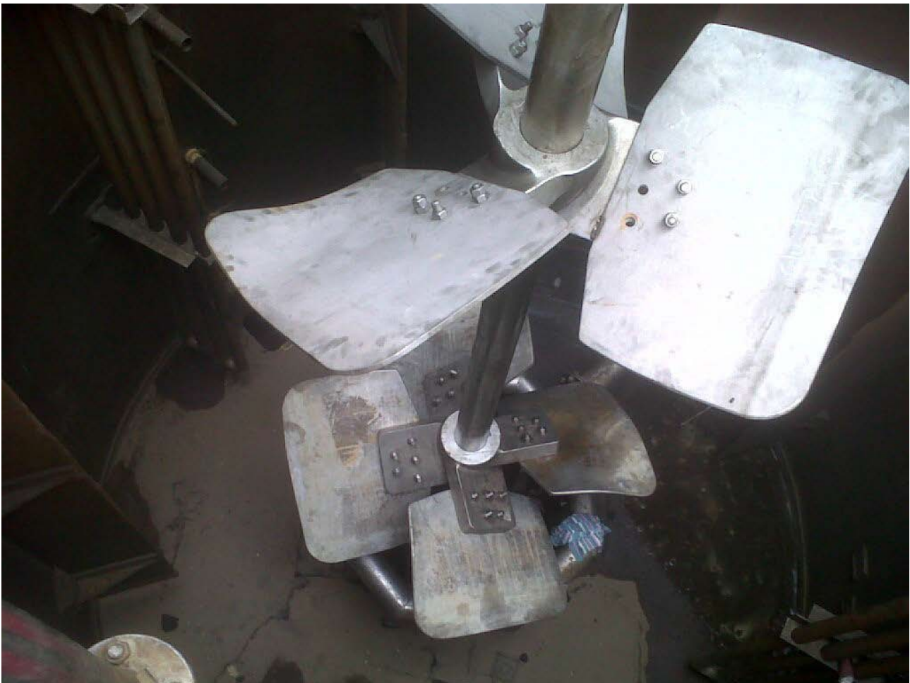
Figure 24: The dual P4/P3 impeller system in the three primary bioleach reactors at the Mondo Minerals nickel sulphide plant (36)
