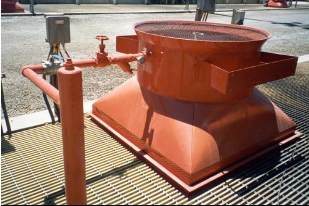
Figure 13. Hi-expansion foam generator installed above one of the trenches in a mixer/settler train. These are initiated by thermal wire detection in the trenches and once initiated can fill the trench of the mixer/settler train affected within a few minutes. The operation of each group of these was tested during commissioning along with the capability to fill the trenches with foam within 2 minutes.
