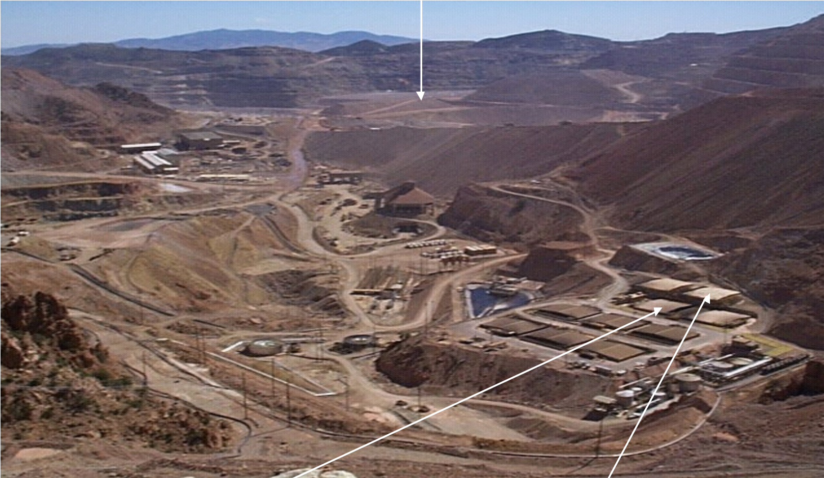
METCALF SX Parallel and Strip Stage Settlers Metcalf SX Facility
