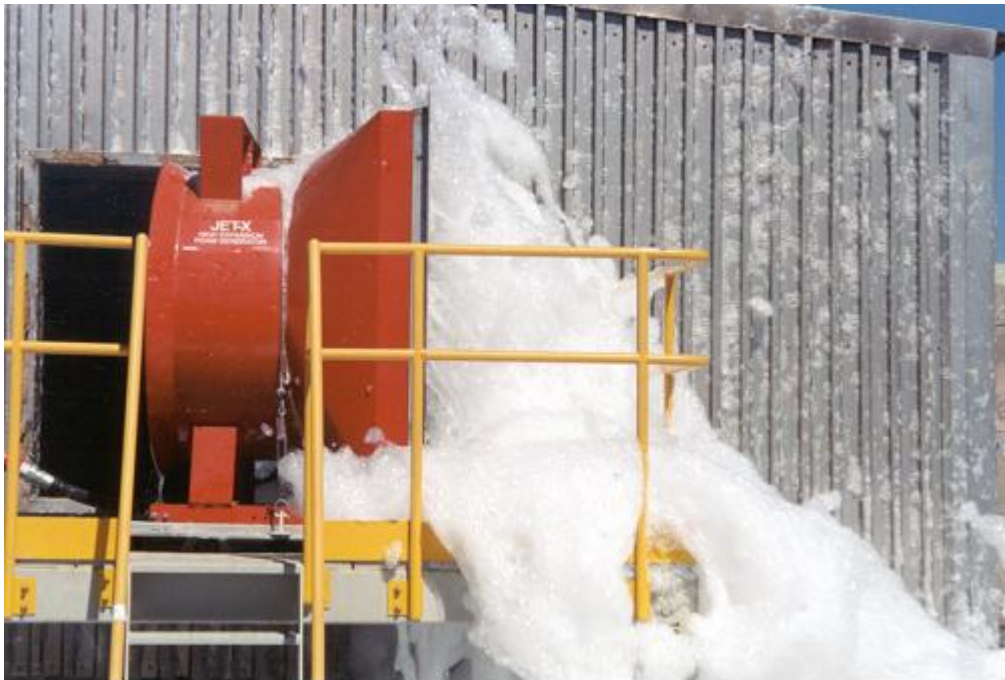
Figure 13. Hi-expansion foam generator installed above one of the trenches in a mixer/settler train. These are initiated by thermal wire detection in the trenches and once initiated can fill the trench of the mixer/settler train affected within a few minutes. The operation of each group of these was tested during commissioning along with the capability to fill the trenches with foam within 2 minutes.
