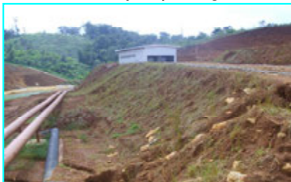
Vetiver grass planted in de-agglomeration and settling ponds
