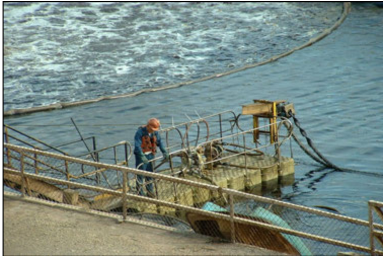
Figure 6: Organic Recovery from Raffinate Pond with a Rope Mop
