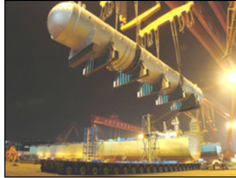
Figure 9 Hoisting of the autoclave
