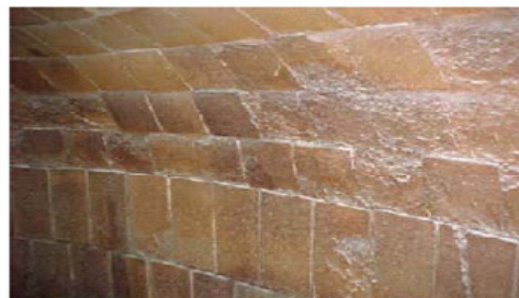
Pieces of brickwork crack when under thermal stress; this is called "Spalling"
