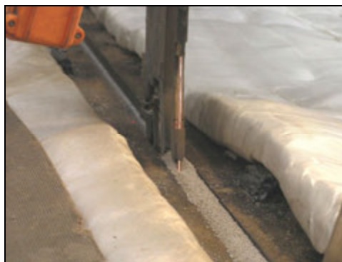
Figure 6: Narrow gap submerged arc welding
