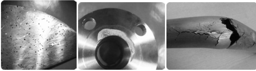
Figure 3: Examples of chloride induce localised corrosion, pitting (left), crevice corrosion (middle) and stress corrosion cracking (right).
