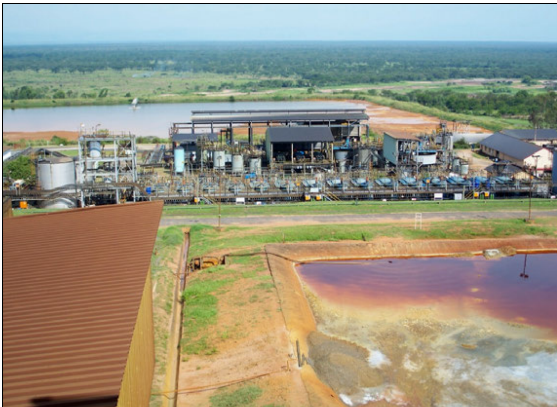
Figure 8: KCCL SX/EW Plant
