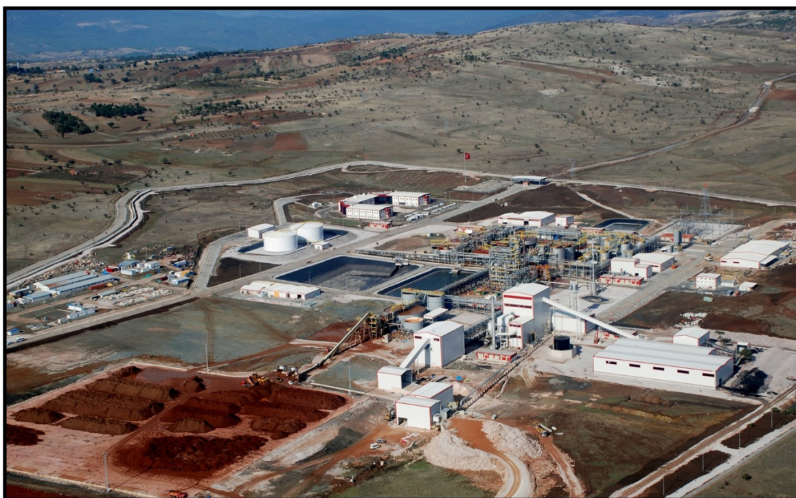
Figure 3 – Gördes Nickel Cobalt Process Plant (Photo courtesy of Meta Nikel Kobalt A.Ş.)
