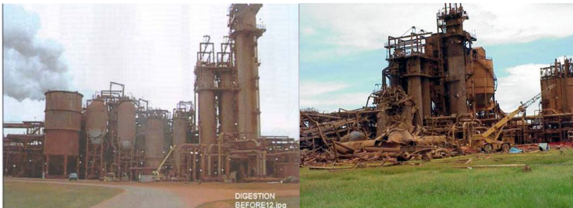
Figure 19 – Gramercy Alumina Plant – Digester Area Before and After Explosion (33)
